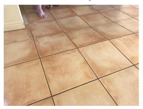
There could be different causes for tiles to become loose, sound drummy or lift altogether over time. These may be related to structural issues with your property, poor workmanship or to other events. Most often drummy tiles are caused by poor tile fitting, structural problems of the floor, or even using the tiled area too early.
