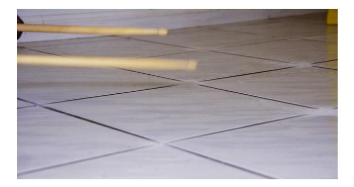
Drummy tiles are loose tiles, which, if tapped with a resonance-testing tool (a metal bar or rod), will produce a drummy type of sound. They are typically detected with ease on floor surfaces, as the latter are subjected to frequent foot traffic. Still, you can get drummy tiles on walls, too.
